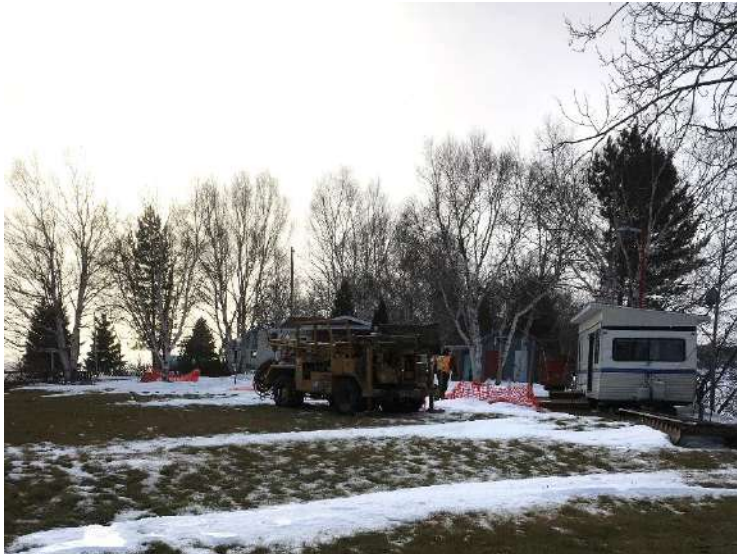
Figure 2-1 Travaux de forages
